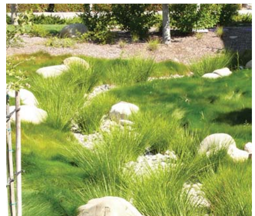
This bioswale, located in San Luis Obispo, was constructed in 2005. Bioswales are an excellent method of Low Impact Design.
